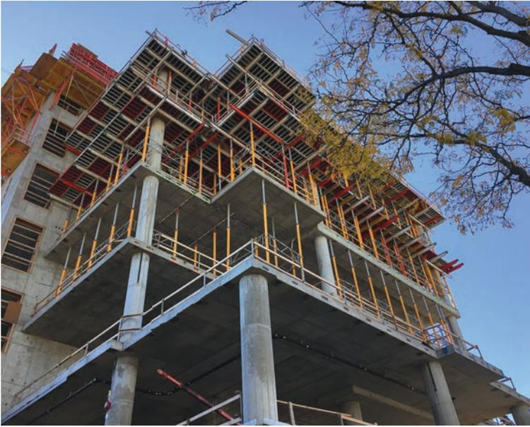
Underside of slabs reveal The Spark's post-tension concrete construction supporting 10 ft (3 m) cantilevered balconies.
