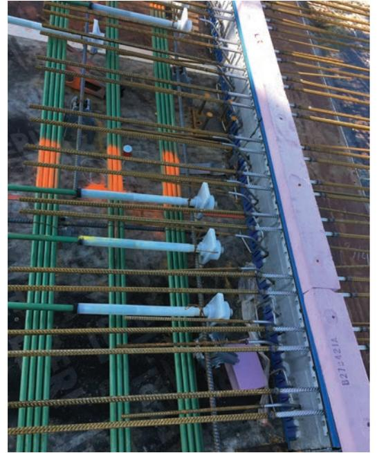
Structural thermal breaks are installed at right angles to the post-tension tendons.
