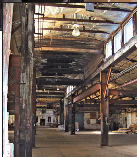
(Top) Paint was removed from the inside brick walls by pressure-blasting them with crushed walnut shells.
